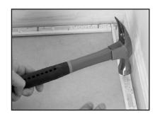
When installing gripper strips on a concrete floor, be sure to use gripper strips with concrete nails (wood nails for wood floors). Ensure that safety glasses are worn when hammering the nails into the subfloor.
