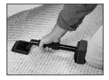
degree angle when kicking the carpet and it should be at the same angle in which you are moving. As you move along the walls, press down on the carpet with your hand behind the kicker head to make sure the carpet sets securely on the gripper.
