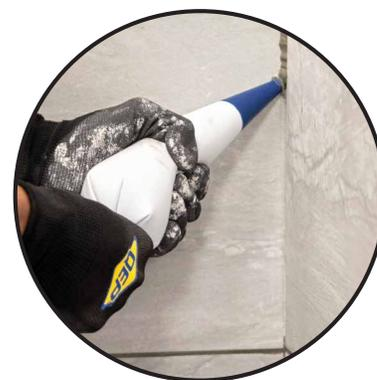
**LA TAILLE DE 32 CM X 58 CM (12<sup>3</sup>/<sub>4</sub>" x 22<sup>3</sup>/<sub>4</sub>" ) FOURNIT UN VOLUME SUFFISANT POUR VERSER LE COULIS RAPIDEMENT SANS RECHARGES FRÉQUENTES**
