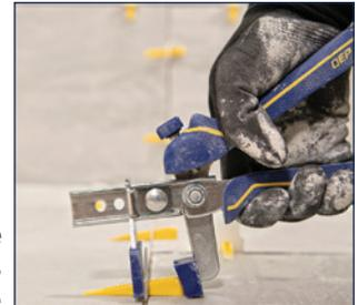
For faster installation use QEP Pro Installation Pliers. See page 10 for details.
