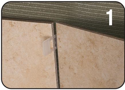
Slide two clips under the tile and into the mortar approximately 2" from each end of the tile. Place the second tile.
