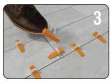
Once mortar has set, simply tap the clips with a non-marring rubber mallet to snap off at the specially designated break-points.
